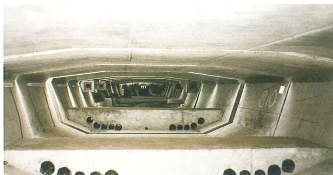
View of deflector beams at centre of bridge span
