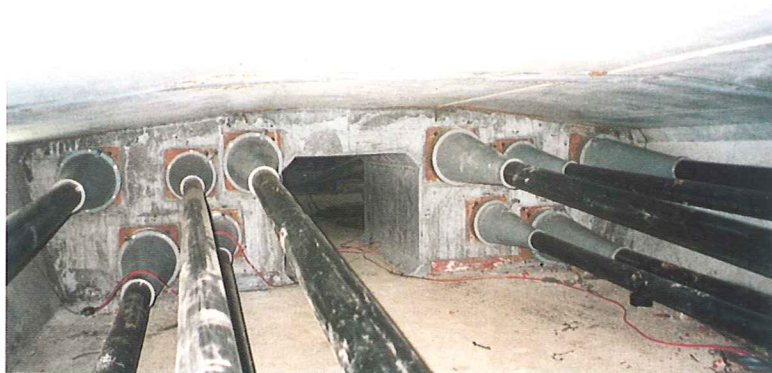
View of coupled and fully stressed external tendons
