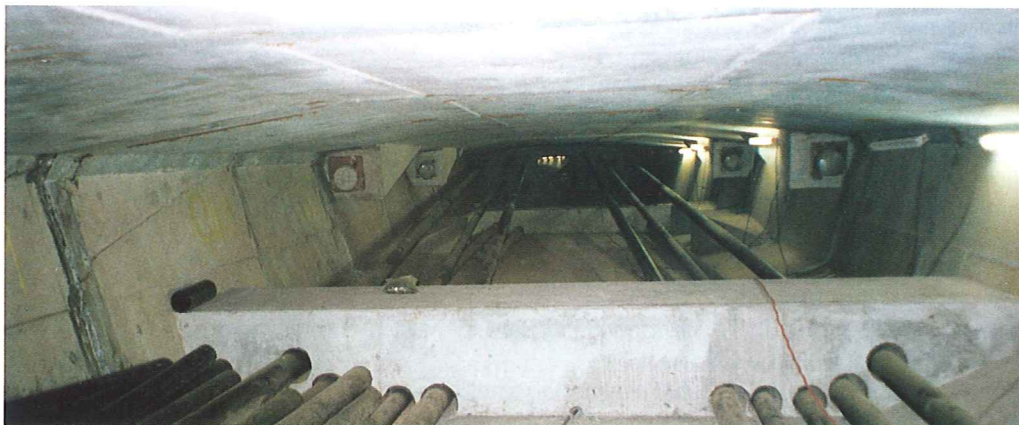
Fully stressed BBR CONA External tendons
