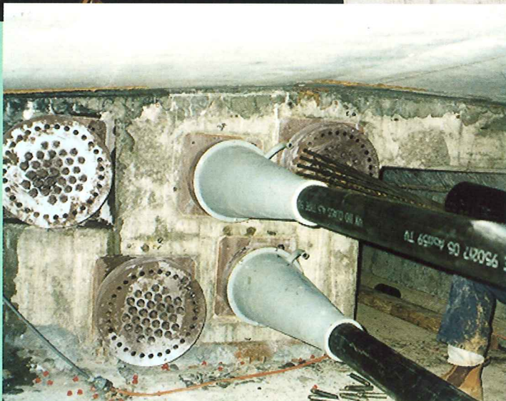
Cables for External Prestressing
