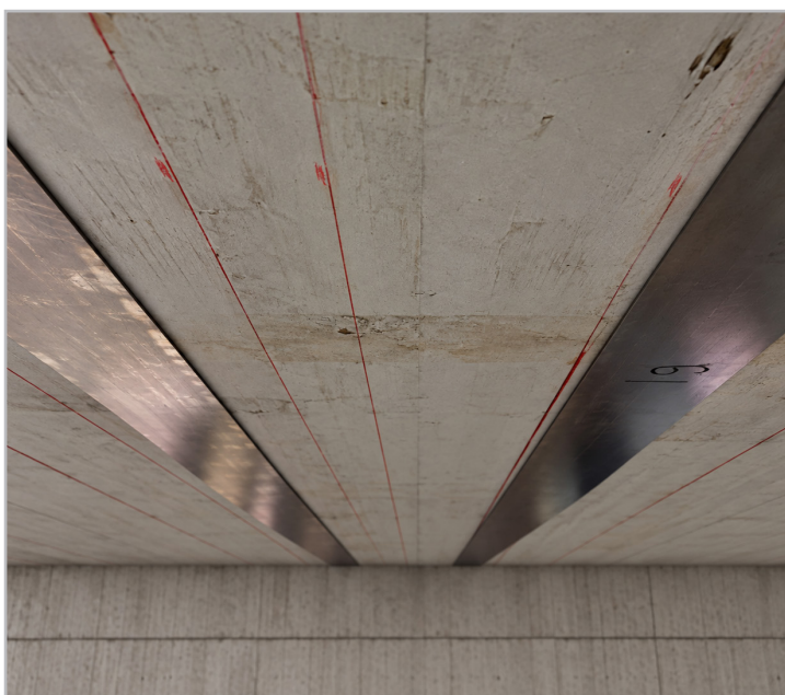
Slab strengthening with CMP-C
