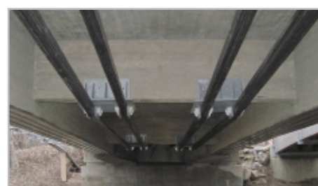
Strengthening from underneath
