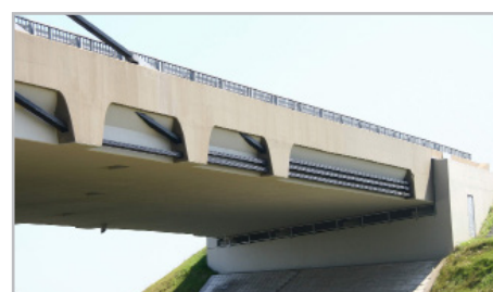
Strengthening along the side
