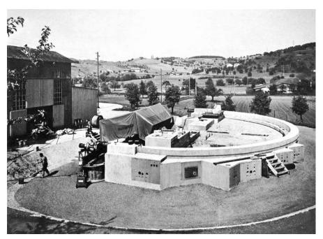
Full-scale installation and tendon replacement test with tendons consisting of strand and wire tendons.
