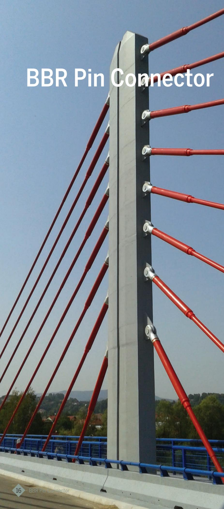
The BBR HiAm CONA Pin Connector is the perfect blend of strength and beauty, while at the same time it extends the inherent benefits of the BBR HiAm CONA family. The BBR HiAm CONA Pin Connector is a beneficial solution for stay cable structures where it is necessary to simplify the end connection detail or to have a certain rotational capability along a specific axis.
