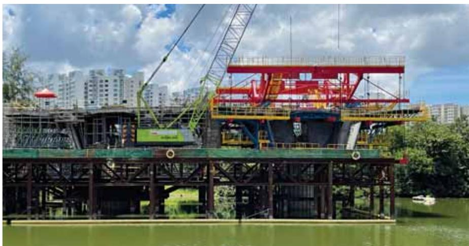
The new Punggol River Bridge in Singapore is taking shape with the help of BBR VT CONA CMI internal post-tensioning to provide the necessary force for the balanced cantilever construction.
