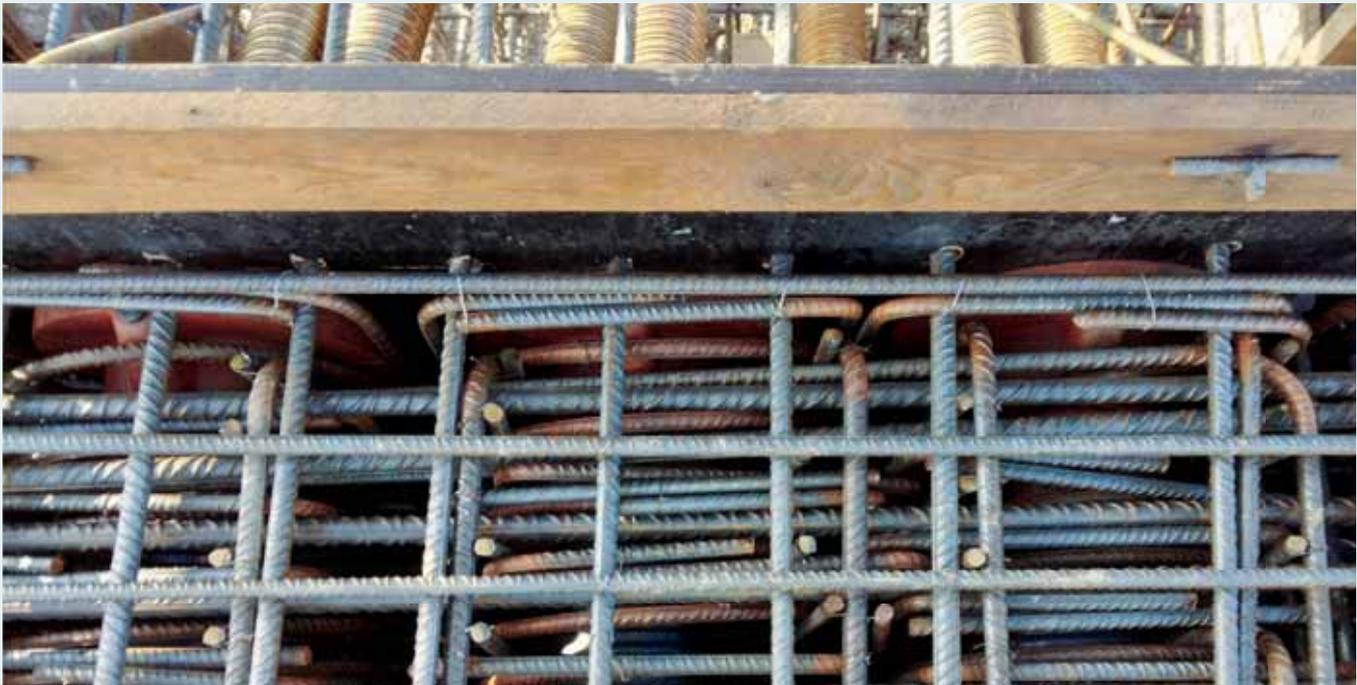
Congestion of reinforcement in the anchorage zone can lead to concrete quality issues and, ultimately, to time and budget overruns.
