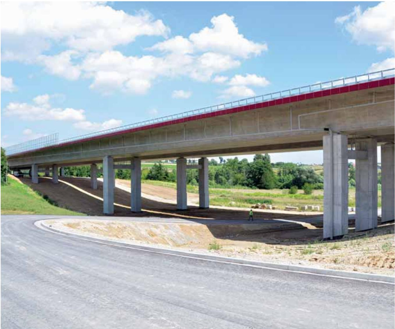
**Our work scope included the post-tensioning of six structures over the new highway and also the post-tensioning and incremental launching of the largest structure on the route ...**
