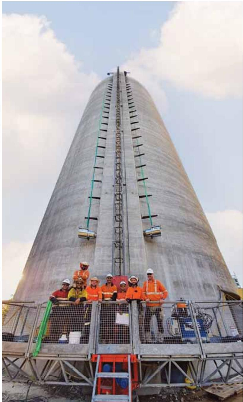
The SRG Global site team celebrate completion of Cement Australia's new 53m high powder storage silo which included CONA CMI internal post-tensioning.
