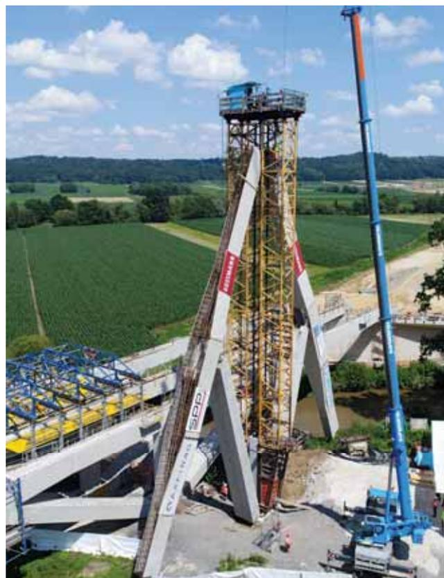
Professor Kollegger's balanced lowering bridge construction method was first applied to the Lahnbach and Lafnitz Bridges, using BBR post-tensioning technology. This innovative scheme was presented with the BBR Network Project of the Year Award 2021 – and a full project overview can be found in CONNECT 2021.
