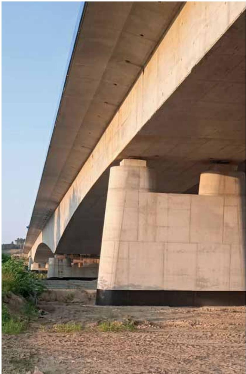
The largest structure on Poland's S19 Expressway, Bridge 08-MS, was constructed using a blended method which included free cantilevering, along with execution of CONA CMI internal and CONA CME external post-tensioning.
