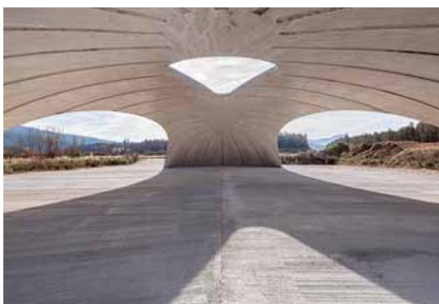
Shell structures: Alternative solutions were needed for filling the voids while creating reinforced concrete double curvature shell structures. Ultimately, pneumatic wedges proved to be the perfect choice. Incidentally, KB VT, the BBR Network Member for Austria, carried out the post-tensioning works for the circumferential tendons during the transformation process from the flat plate to the shell structure. The smaller shell received a 'special mention' at the 2018 *fib* Congress in Melbourne.
