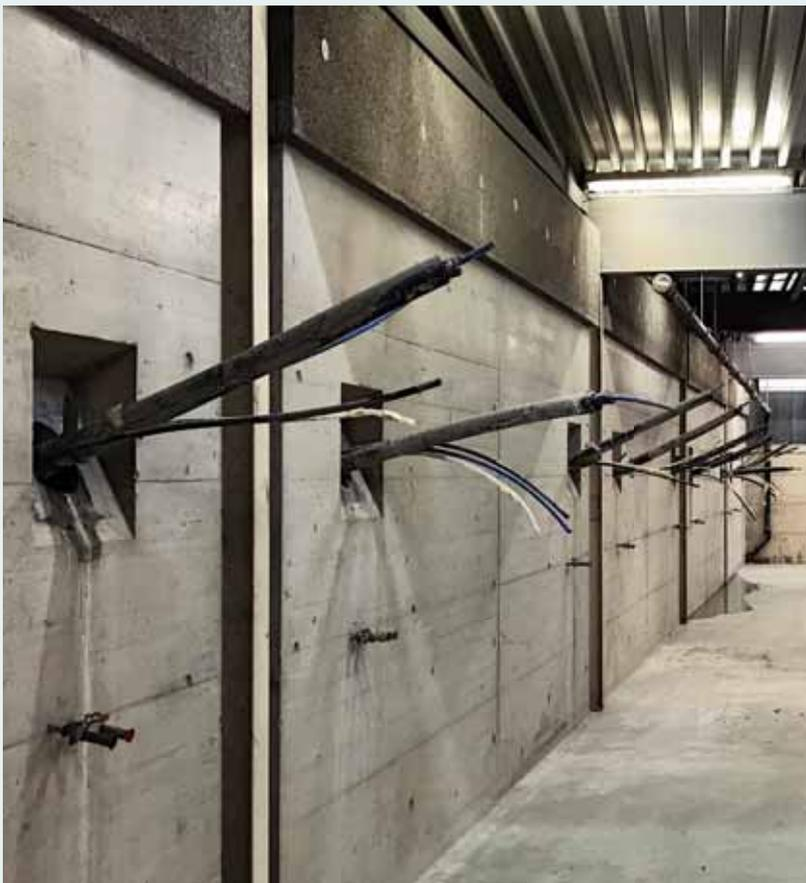
Strand ground anchors play a critical role in retaining and prolonging the life of major structures, such as this underground car park in Switzerland. Photograph courtesy of Stahlton AG.
