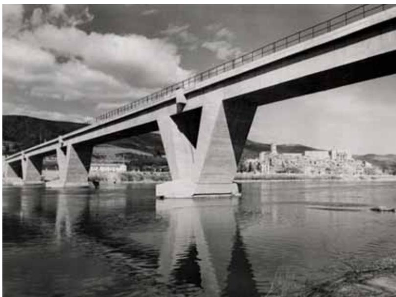
At the time of its construction, back in 1952, the La Voulte Viaduct in France was the world's longest prestressed precast segmental bridge – and it featured BBR post-tensioning technology.
