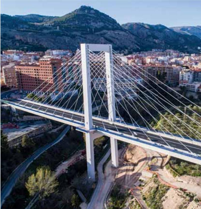
Fernando Reig Bridge, Spain – a stay cable replacement project requiring an innovative destressing technique was carried out by Spanish BBR Network Member, FCC Construcción, S.A.
