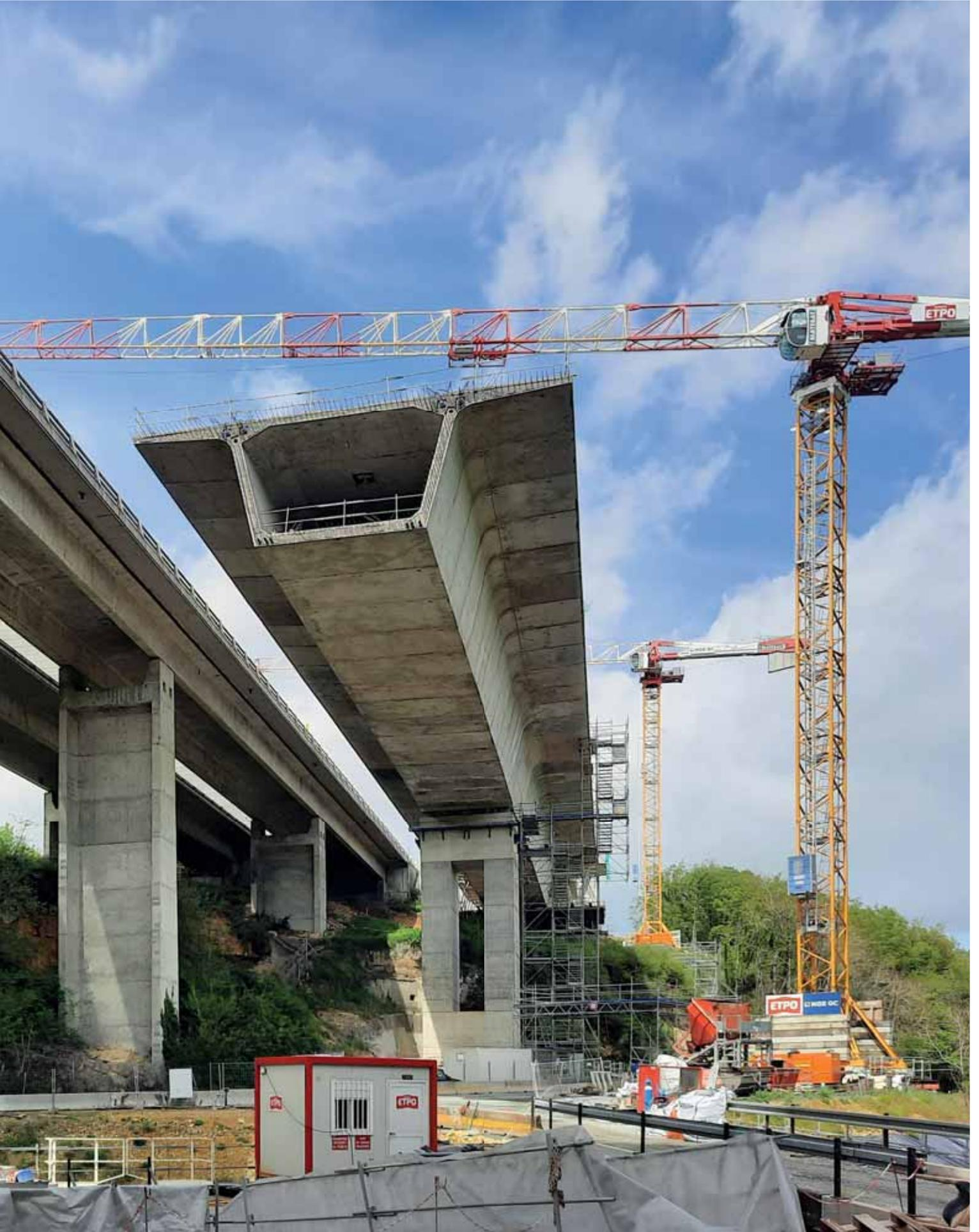
A great technical solution is being delivered to increase motorway capacity here in the Touraine region. The widening of the A10 motorway involves the construction of a third viaduct, to carry an additional two traffic lanes plus an emergency lane, alongside the two existing structures.
