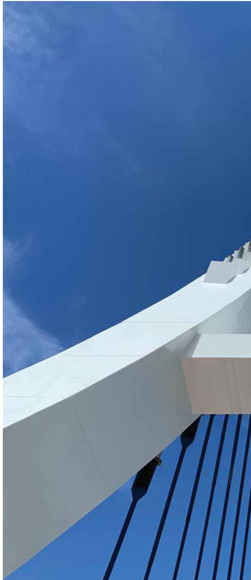
A total of 27 pairs of BBR HiAm CONA stay cables were installed for the bridge.
