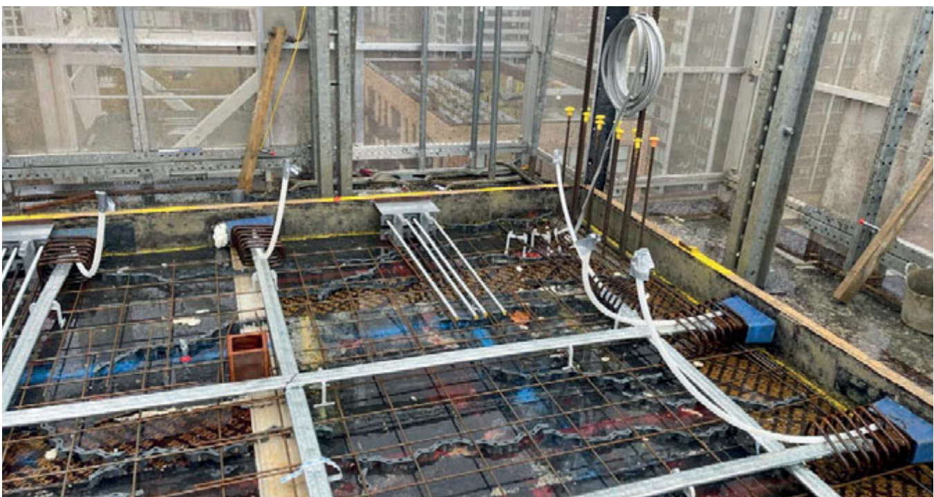
PT installation underway at Elephant Park, a sustainable high-rise development in London.
