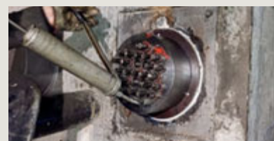
Applying grease to seal the tendon and to enhance corrosion protection.
