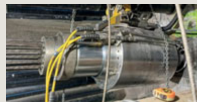
Post-tensioning using jacking equipment to apply precise tension to the tendon.
