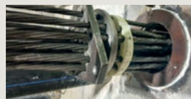
Positioning the tendon with the anchoring device during installation.
