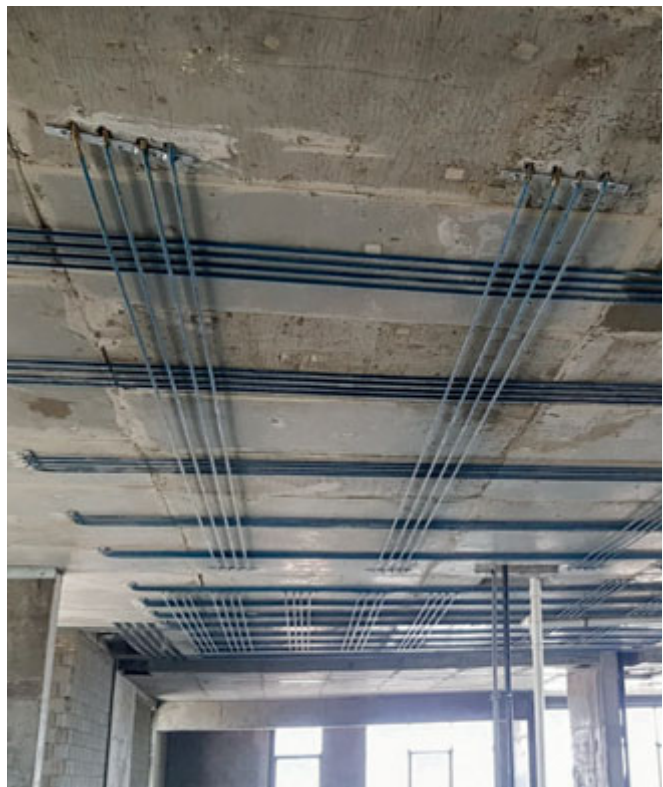
BBR Care+ in action: an existing hotel in Saudi Arabia was transformed into the Khurais Hospital, upgrading structures for the higher loads of hospital beds and equipment, rather than demolish and rebuild.
