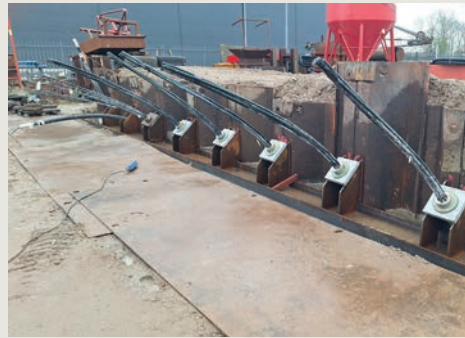
Multiple ground anchors installed along a sheet pile retaining structure, showing the repeatability and technical discipline of specialist anchor works.
