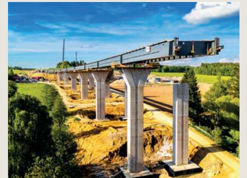
Bridge construction on the D3 Kaplice–Nažidla project, illustrating MI Roads' role in major Czech transport infrastructure works.
