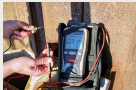
Electrical resistance measurement during anchor inspection, supporting durability control and performance verification on site.
