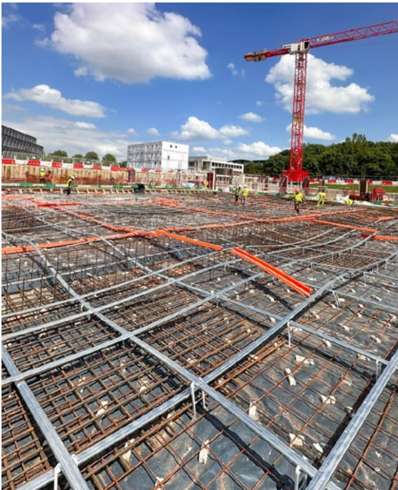
Post-tensioning installation underway at The Oxford Science Park expansion.
