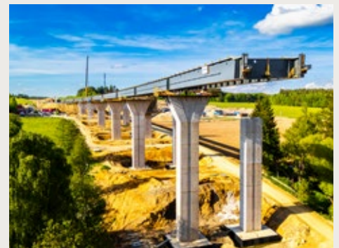
Bridge construction on the D3 Kaplice–Nažidla project, illustrating MI Roads' role in major Czech transport infrastructure works.
