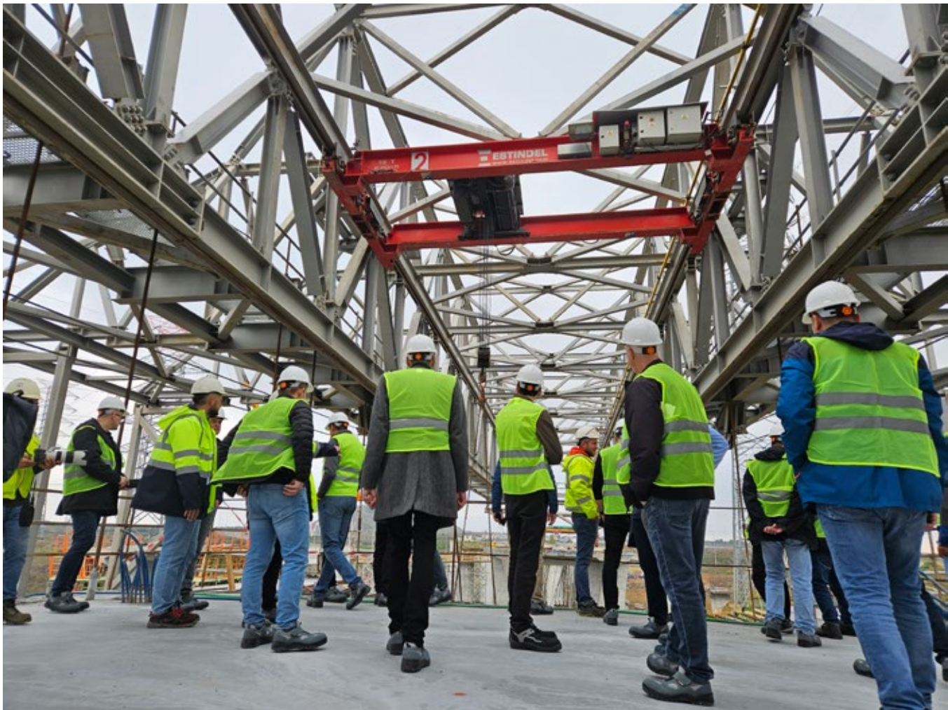
BBR Global Conference and BBR Training delegates visiting the Sular Valley Viaduct construction site.
