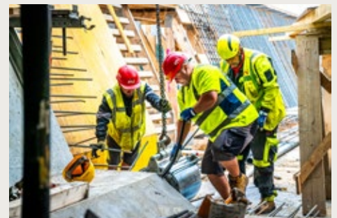
Site teams working with bridge prestressing equipment, highlighting the practical engineering capability behind MI Roads' specialist operation.
