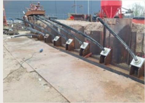
Multiple ground anchors installed along a sheet pile retaining structure, showing the repeatability and technical discipline of specialist anchor works.
